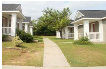
Exterior After Renovation
