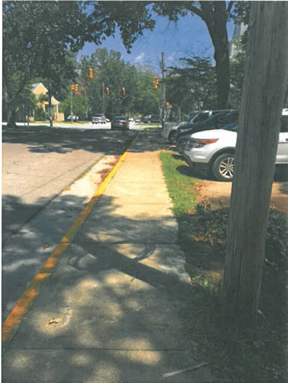
Existing curb cut facing northbound on Sims Avenue
