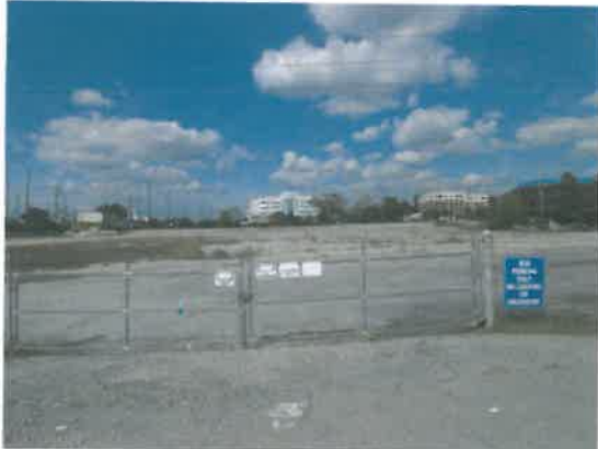
1 LOOKING NORTH FROM THE MIDDLE OF WASHINGTON ST.
